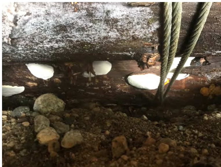
Top layer of stringers condition
