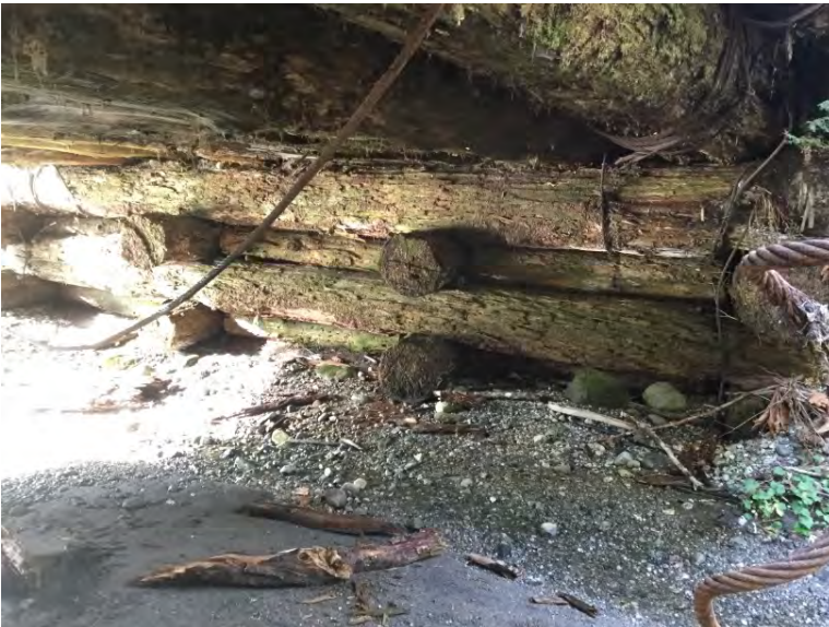
Right Bank Abutment when facing downstream
