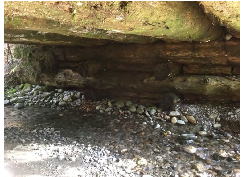
Left Bank Abutment when facing downstream
